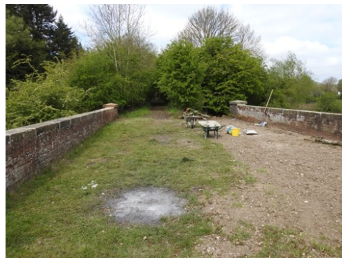
Bridge 1714 after removal of excess spoil and vegetation.
