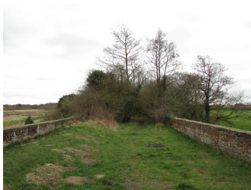
Bridge 1714 before work started.
