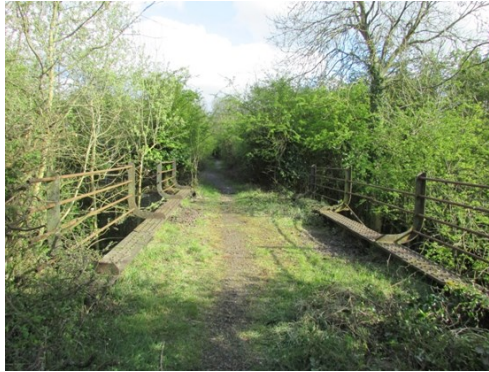
Bridge 1715 over the M & G N track bed before work started.
